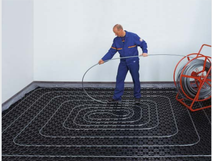
Fig. 10: Installing an underfloor heating/cooling system
